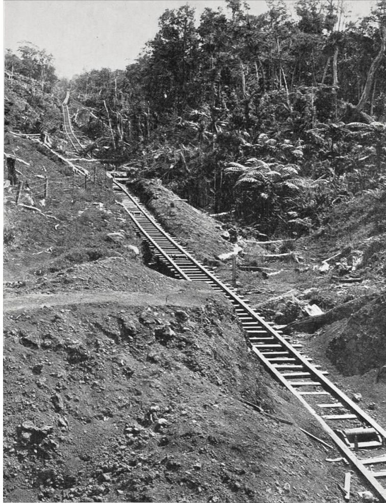
ABOVE: THE STEEP TRAMLINE ON WHICH TIMBER IS BROUGHT FROM THE SIBERIA BUSH KAIHU 6
