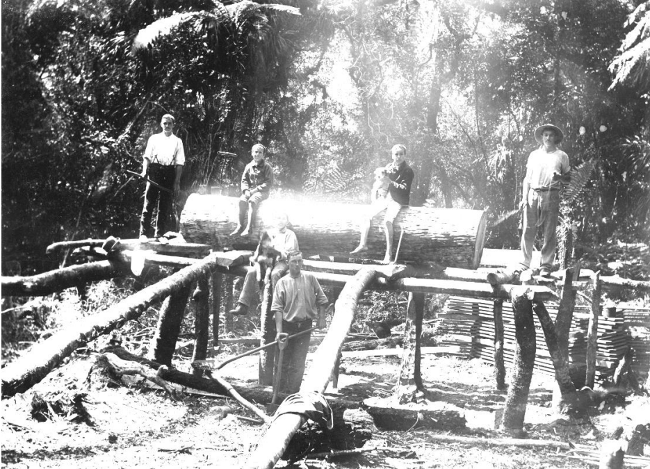
LEFT: SOME OF MY RELATIONS PIT SAWING TIMBER IN THE WAIKATO
