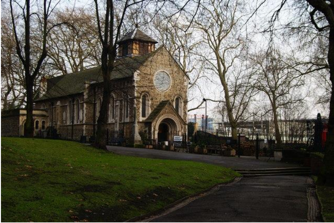
ABOVE: SAINT PANCRAS OLD CHURCH PANCRAS ROAD LONDON
